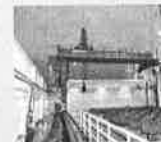
Riser handling crane
